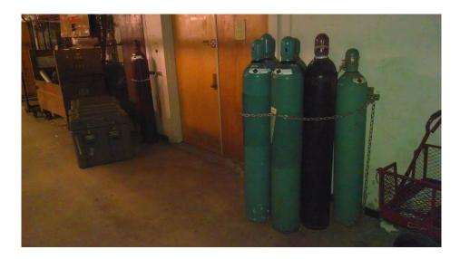
Lastly, what are the exposures? Although they are properly secured, these hydrogen and oxygen cylinders are directly in the vicinity of the electrical area and present exposure hazards in themselves.
