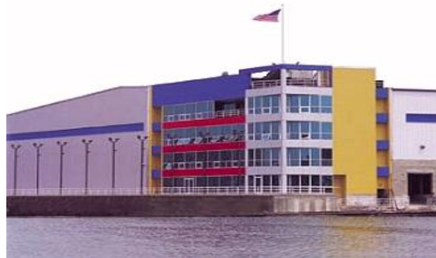
Citi-Storage photo courtesy of Google Earth.
