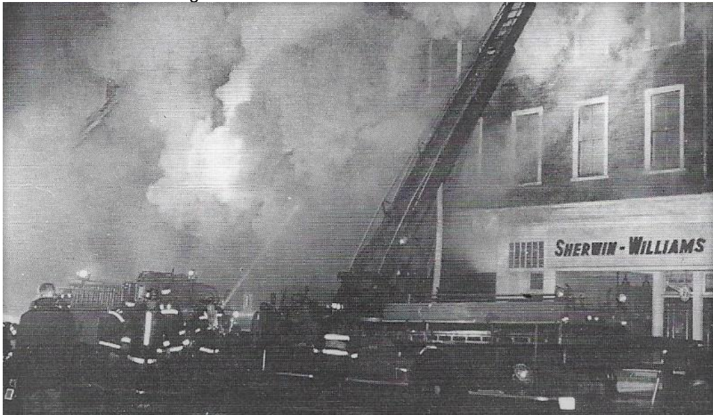
Front of the building after transmission of the third alarm. Photo by Ray Barnes
