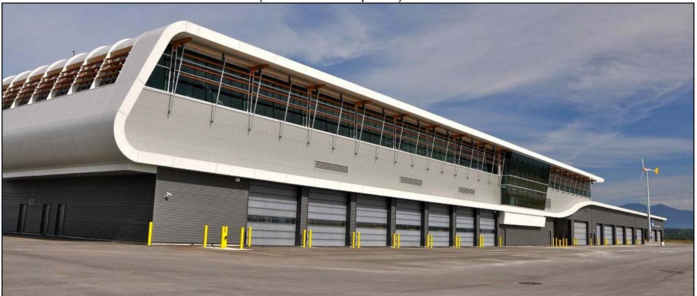
Vancouver Airport's massive new fire station has seven bays, with the remaining doors for mechanical work and seasonal vehicle storage. The two story section used by fire opened in June after a major retrofit. Aside from the usual crew quarters on the ground floor, there is a separate decontamination shower/change area, material storage (Terry counted 250 50lb pails of purple K and a foam tank that measures 12'x12'x10', the latter equipped with a pump and hose for easy refilling). Also on ground level are incident debriefing rooms, offices and a room for testing and filling extinguishers. Upstairs are a boardroom, exercise room, a large kitchen and dining area, more offices and an open patio for the crews to relax in. (Info & picture from Terry Yip)
