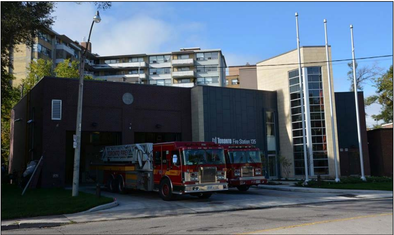
Toronto Fire Services newest hall in Forest Hill. Station 135, located at Chaplin Cres., is only the second building to house this company since the old Forest Hill VFD was created almost 100 years ago. It's much larger than the old premises and features a LEED certification and underground parking, a first for the TFS. It went into service September 30. (Larry Thorne photo)
