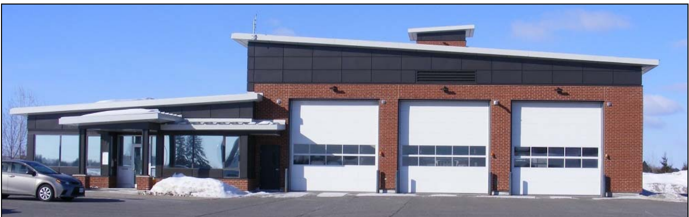
Ottawa's newest hall opened in the winter. Station 73 is located at 6090 Rockland Rd. in Vars. It's a volunteer station housing a pumper-tanker, tanker and support unit. (Ken Walton photo)
