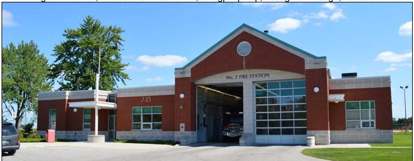
Also seen on the tour was St. Thomas Station 2, at 235 Burwell Rd. Built in 2006, it houses two pumps. (Rick Loiselle photo)
